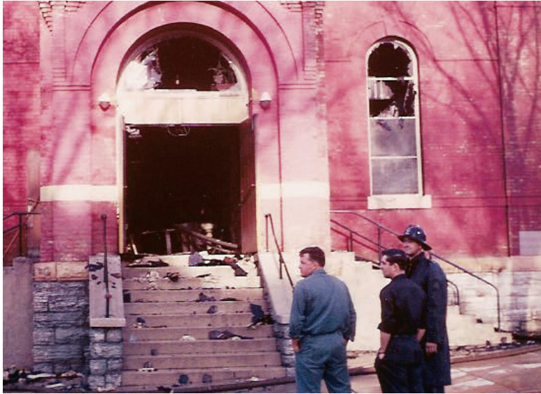
Exterior of the main entrance after the fire.
