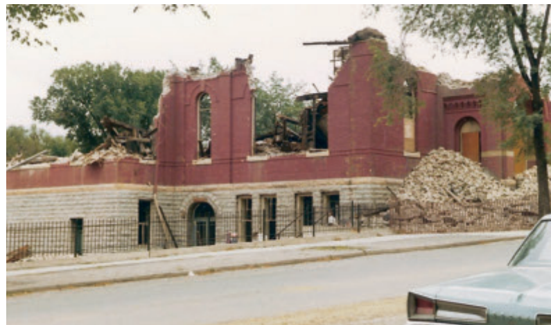
TOP: The interior of the church after the fire including the altar area, choir loft and main church entrance.
